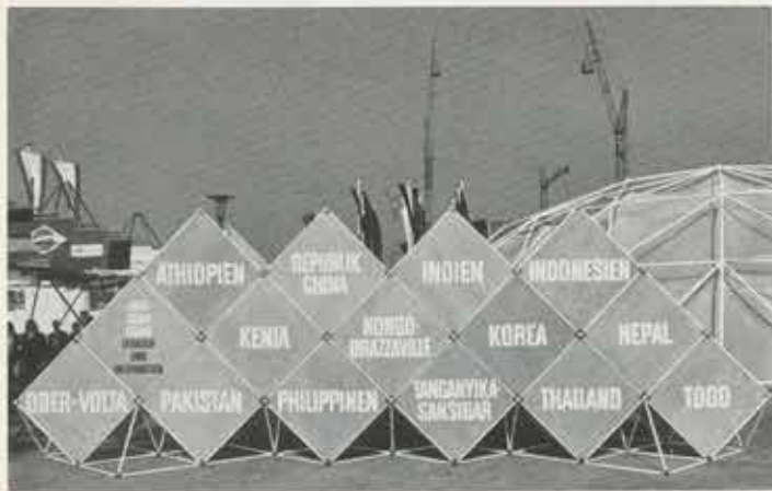
9. The display units inside the tents were composed of "Mero" standard components, forming octahedrons and tetrahedrons. In the foreground, a combination of table and glass pyramids; in the background, a number of target units.
